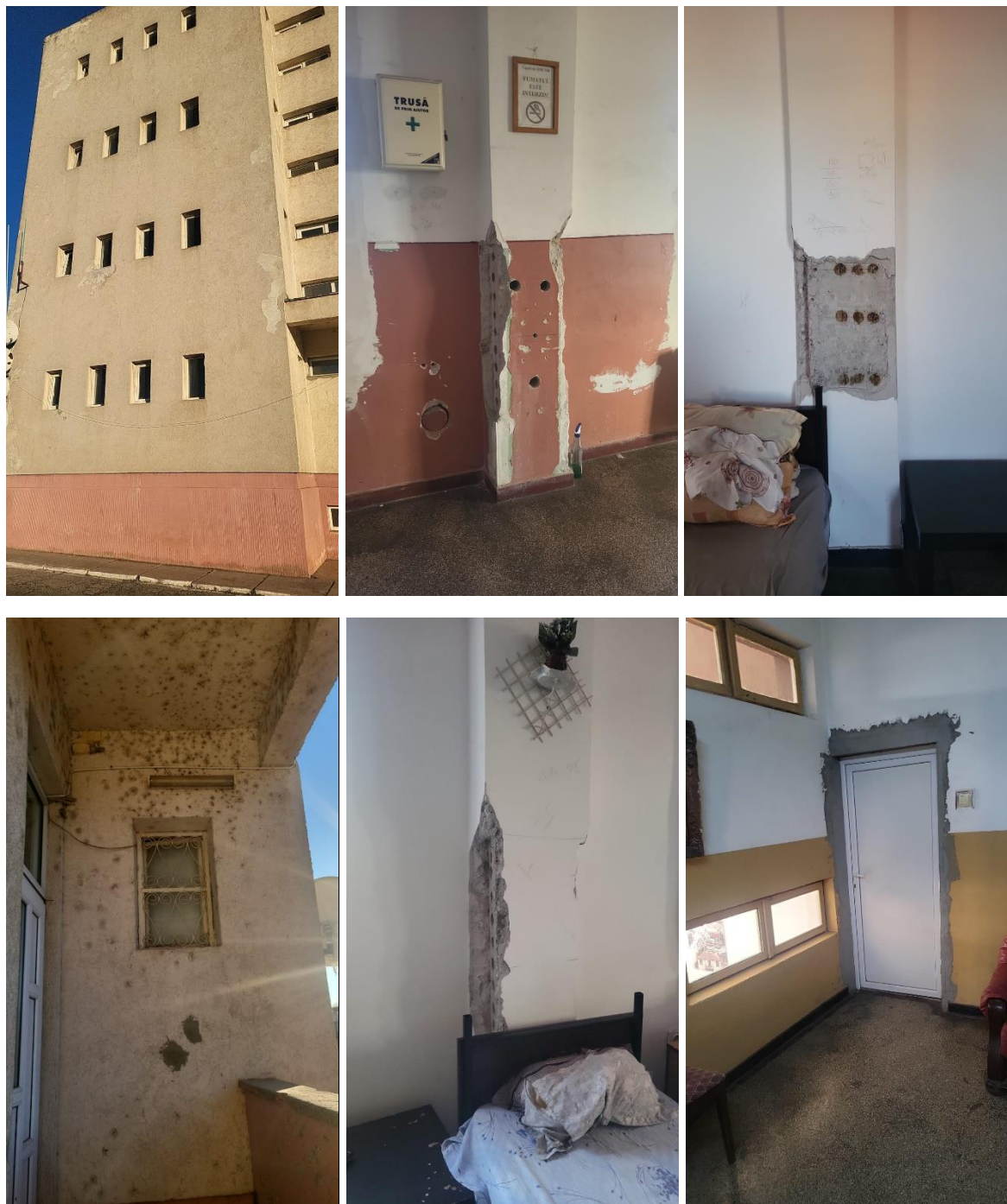
Figure 6 Existing CPF D's C1 administrative building
